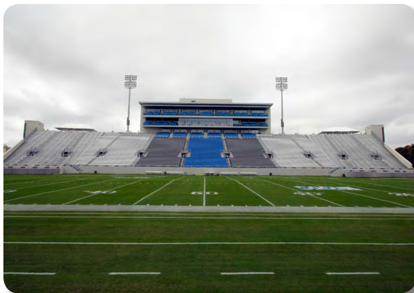
Johnson Hagood Stadium
